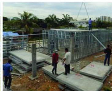
Precast Half Slab
