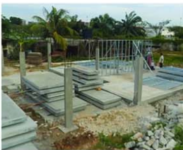
Ground Floor Wall Frame
