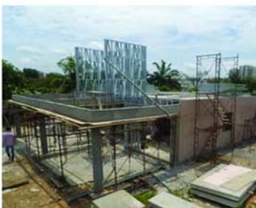
First Floor Wall Frame
