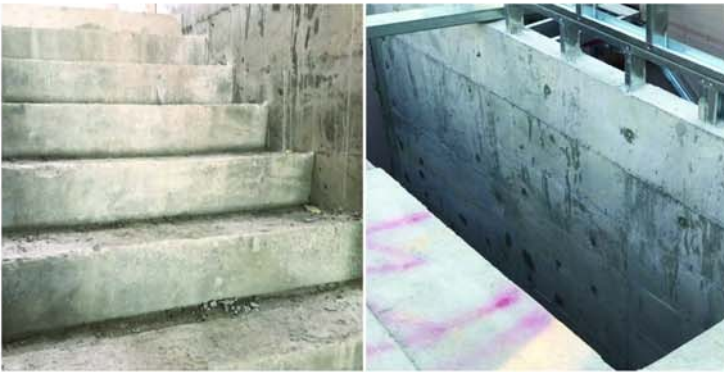
Staircase after casting
