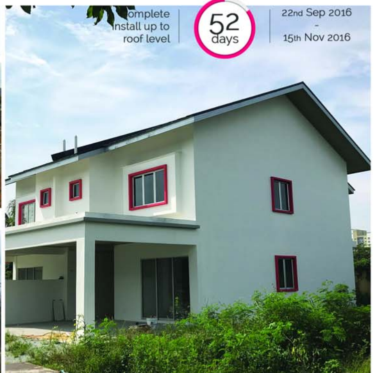
Completion of Works Up to Roof Level
